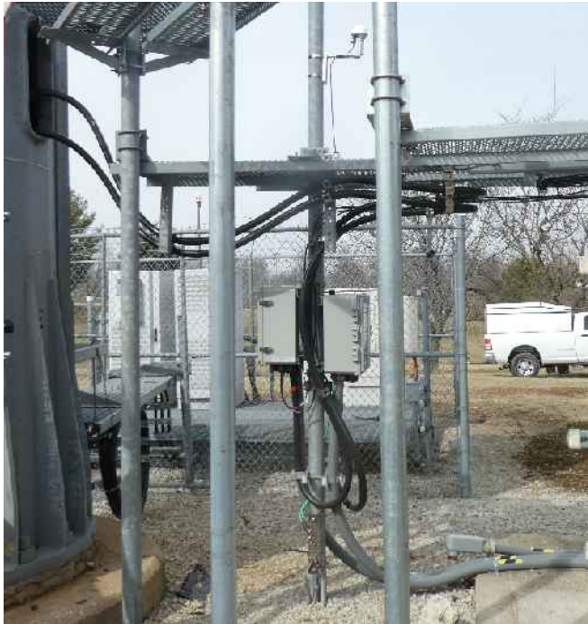
G EXIST. CABLE ROUTE SCALE: NONE
